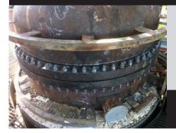
**OMV Petrom Romania site required our assistance to install a critical gasket during a major shutdown**. Our engineer supervised the entire installation of a specially designed Thermiculite<sup>®</sup> Kammprofile on the main reactor flange, resulting in a leak free start up on a critical vessel during a major shutdown, which enabled the site to meet industry best practice according to ASME PCC-1-2013.
