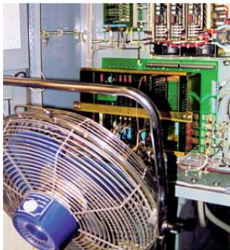
A dangerous shock hazard exists when the panel door is opened to let a fan blow hot, dirty shop air at the electronics.
