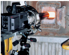
Special high temperature vortex tubes keep a boroscope lens cool while inserted into a 1200°F boiler porthole.
