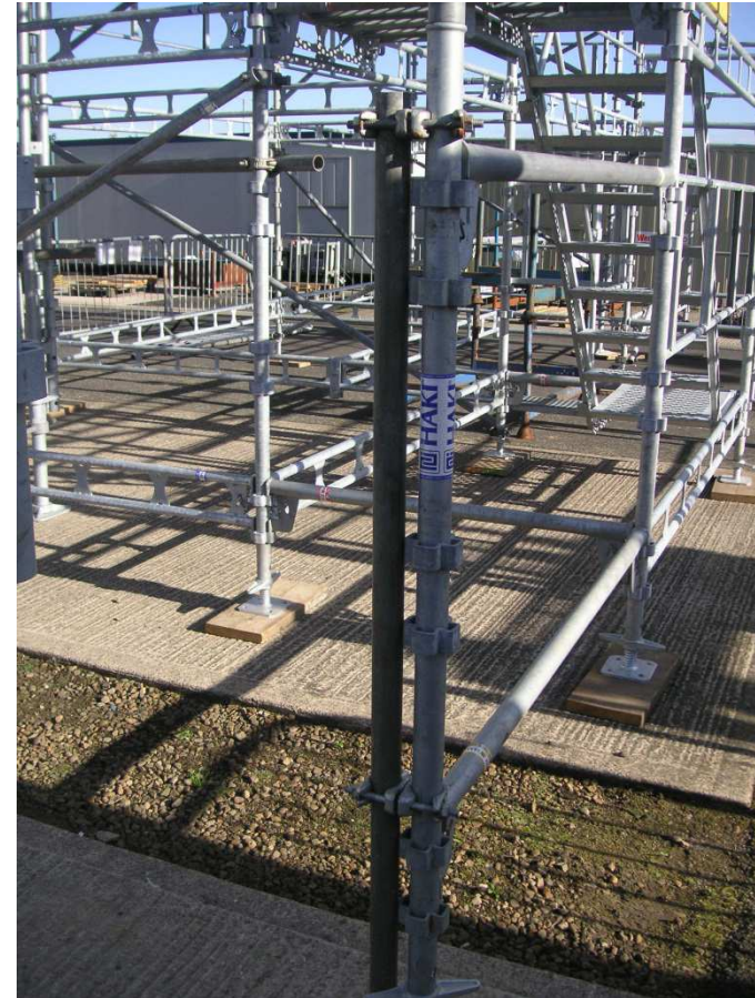
Splicing with standard couplers
