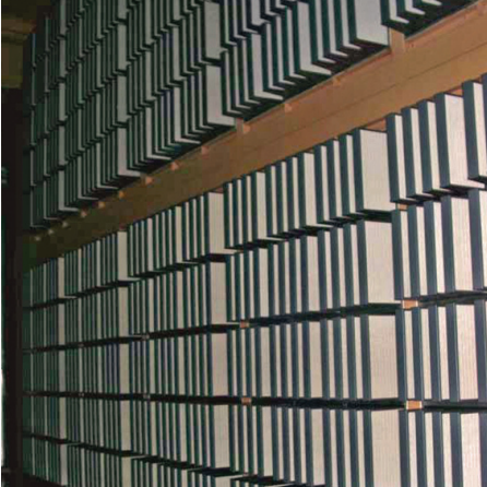
◀ Compatex TMPC filters installed at a gas turbine power station
