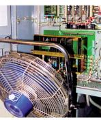
A dangerous shock hazard exists when the panel door is opened to let a fan blow hot. dirty shop air at the electronics.
