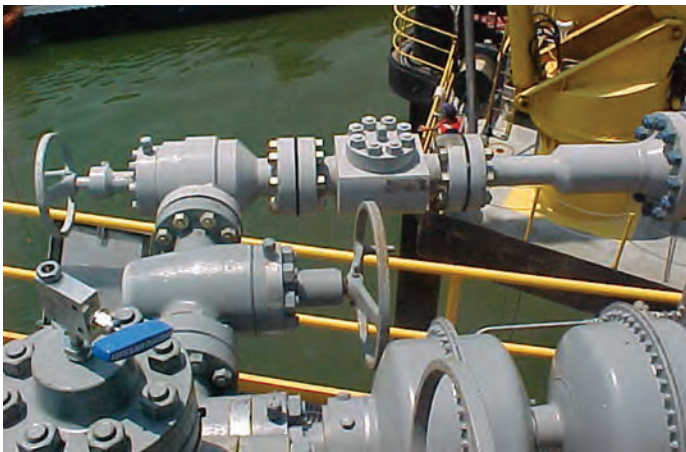
PRS installed within a flow line
